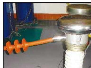
22kV 1-core outdoor termination is under testing
